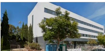
Fig. 2 Construction of CE 2 (Autor)
